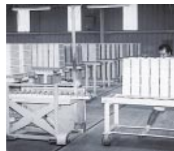
Roller conveyors on a cart and scissors lift—replaces lifting and carrying with rolling and sliding
