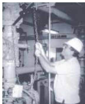
A pull chain makes opening the valve easier
